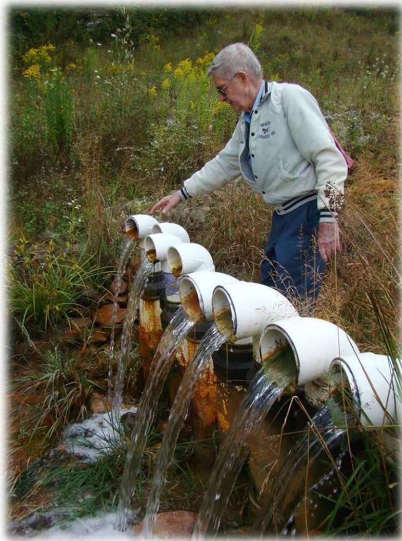
Figure 194 – Thurman Korn explains the Moore No. 7 treatment system
