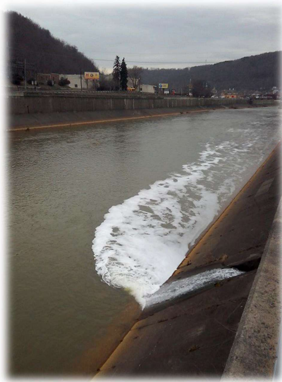
Figure 28 – A permitted point-source discharge, associated with the Cambria Iron Stormwater NPDES permit, enters the Conemaugh River in Johnstown (Lazzari)
