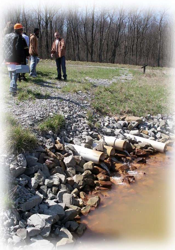
Figure 202 – Students tour the AMD treatment system at Keystone State Park
