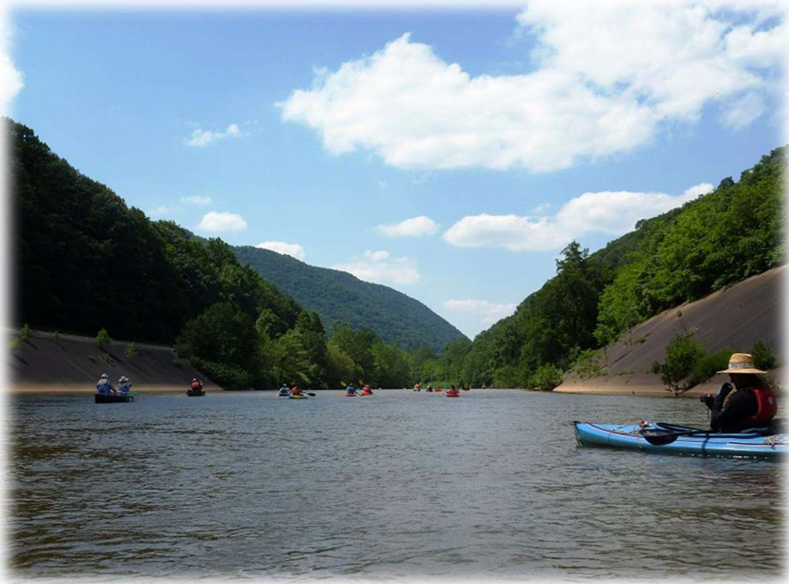
Figure 57 – Participants in the CVC’s Stony-Kiski-Conemaugh River Sojourn paddle the Conemaugh River through the Conemaugh Gap. Note the end of the flood walls
