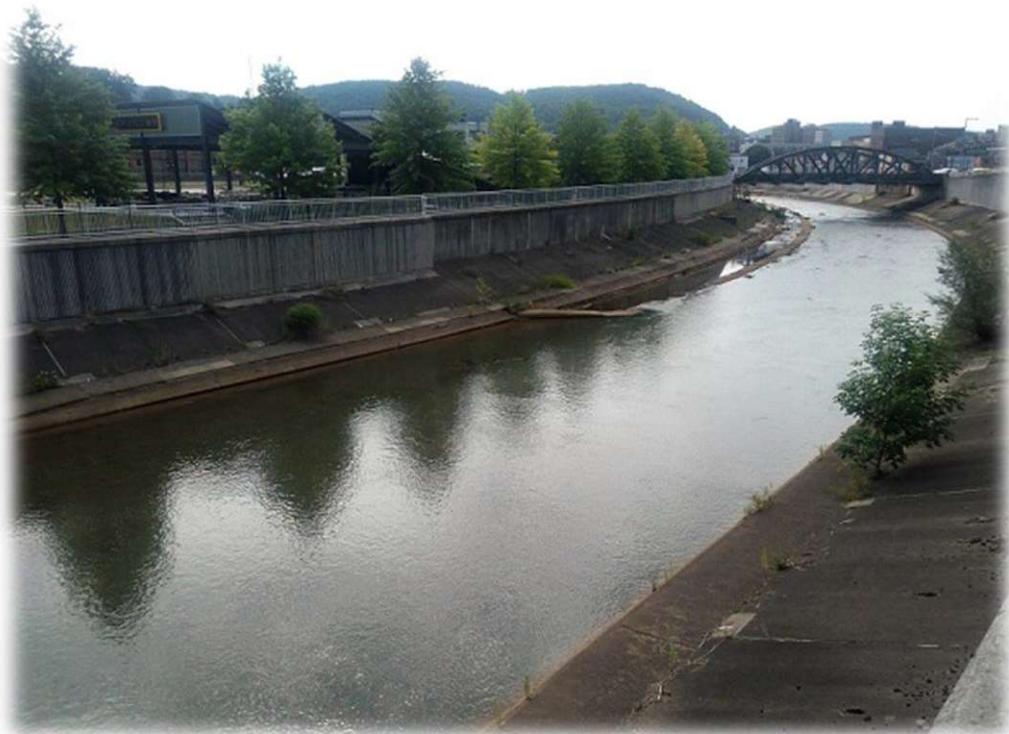
Figure 35 – Johnstown's floodwalls as seen along the Little Conemaugh River
