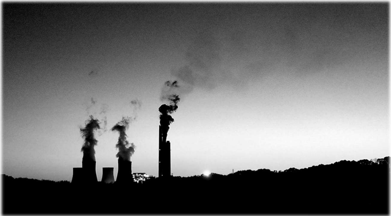
Figure 25 – Keystone Generating Station at dusk
