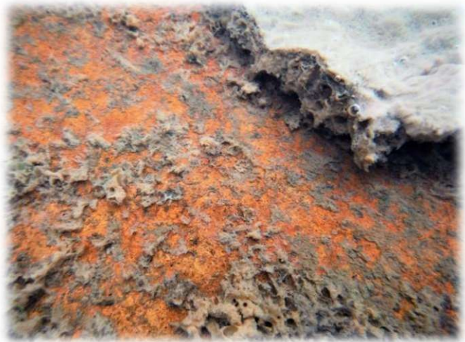
Figure 137 – A close-up of the armoring in Yellow Creek below the treatment systems
